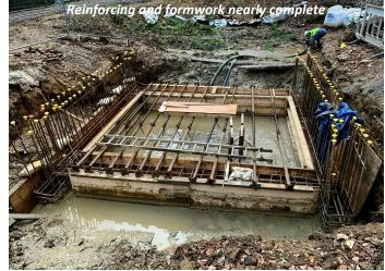
work panels (made by Martyn Baker and Len Hasler at the Tickner's depot). So, with the formwork virtually complete, the first concrete pour can go ahead, which will, because of the location of the project, be quite unique! But more about that next month.
