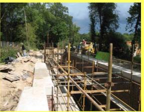
Recent work at Southland sees the lock chamber nearing completion, with all brickwork now finished and work concentrating on the copings and training walls, ready for the gates which are now on order (Eric Walker)
