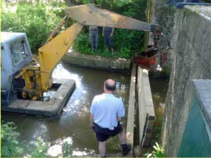
Above and right: The Monday (Mrs Bucket) group installing stop planks at Baldwin's Knob Lock as part of the recent emergency repairs to a gate (pictures by Martin Burgess)
