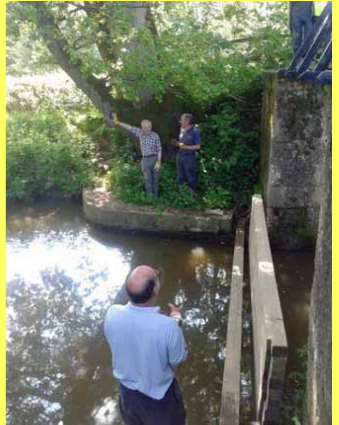
Above and right: The Monday (Mrs Bucket) group installing stop planks at Baldwin's Knob Lock as part of the recent emergency repairs to a gate (pictures by Martin Burgess)
