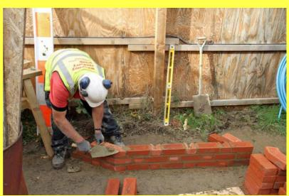
London WRG's October visit: (top) building a bund across the canal so that the water level can be lowered, plus new pipe; (above) Martin with a trial panel of Flemish bond brickwork; (leftt). excavations to find the water pipe, we have agreed with Thames Water that we can reduce costs if volunteers can prepare the trench. Pictures from Sally Schupke
