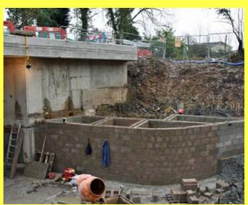
Compasses Bridge - the south western wing wall. The concrete blocks form the shuttering for the structure which will be filled with concrete. The outside surface will be clad with facing bricks. (Photo: Dave Verrall)
