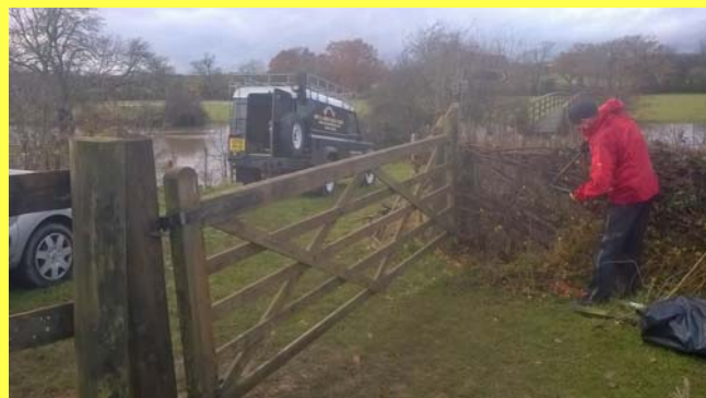
The rebuilt gate and fence at Haybarn (Martin Burgess)
