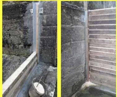
Stop plank channels and stop planks at Drungewick (Kev Baker)
