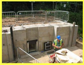
Lock HS Sluice Blade & Connecting rod being installed
