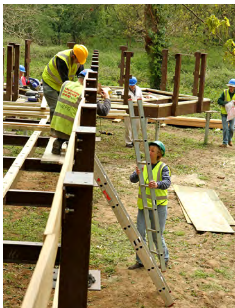
Above left: working party leader George Whitehead installing the timber frame for the Hunt Park Viewing Platform. Above right: a team of skilled carpenters was supported by others who helped with less demanding jobs. Below: the hexagonal shape of the platform meant a tricky construction task. (Mike Hobbs)
