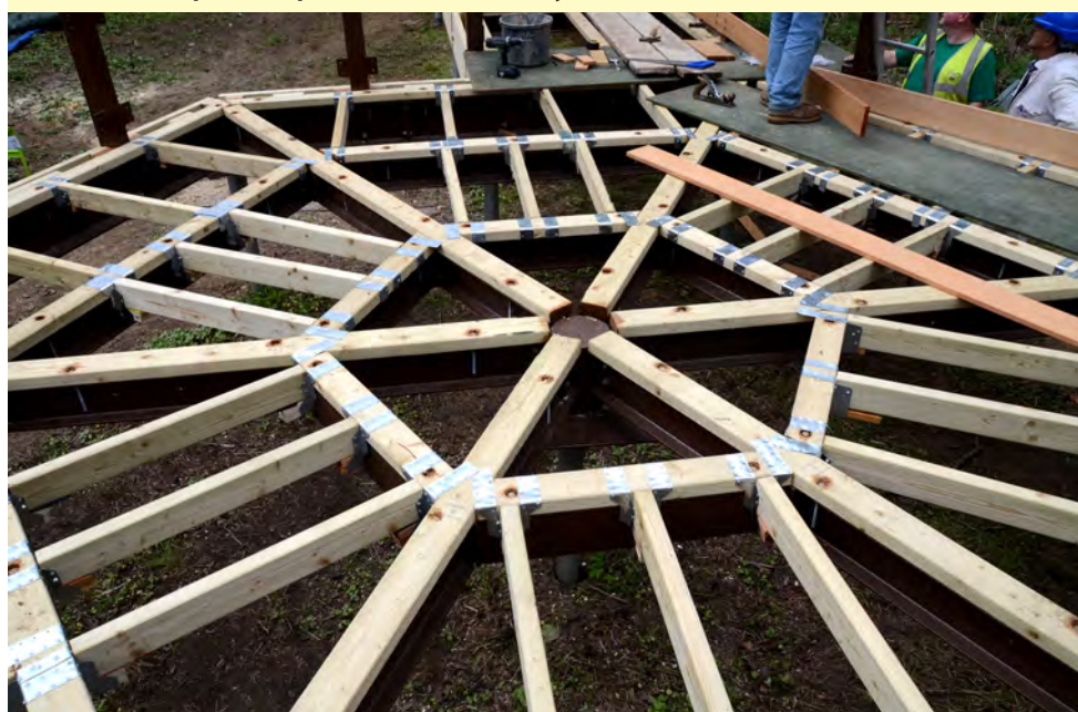
Above left: working party leader George Whitehead installing the timber frame for the Hunt Park Viewing Platform. Above right: a team of skilled carpenters was supported by others who helped with less demanding jobs. Below: the hexagonal shape of the platform meant a tricky construction task. (Mike Hobbs)
