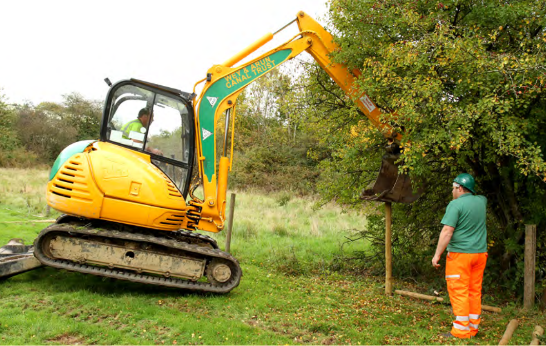
Above: That's one way to knock in a fence post - Andy Evans (driver) and Dave Evans with the Summit Working Party at Tickner's Heath. (Julian Morgan)
