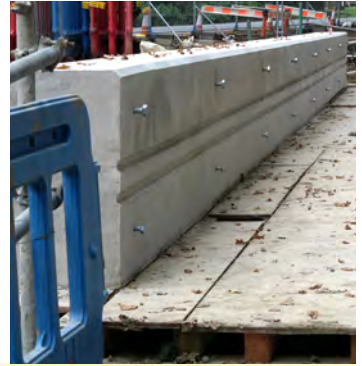
Left: The wooden parapets on the new Compasses Bridge will be similar to those used on this bridge across the River Wey at Tilford in Surrey. Right: Bolts installed in the concrete sides of the new bridge deck ready to take the parapets
