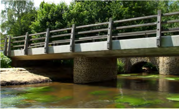
Left: The wooden parapets on the new Compasses Bridge will be similar to those used on this bridge across the River Wey at Tilford in Surrey. Right: Bolts installed in the concrete sides of the new bridge deck ready to take the parapets
