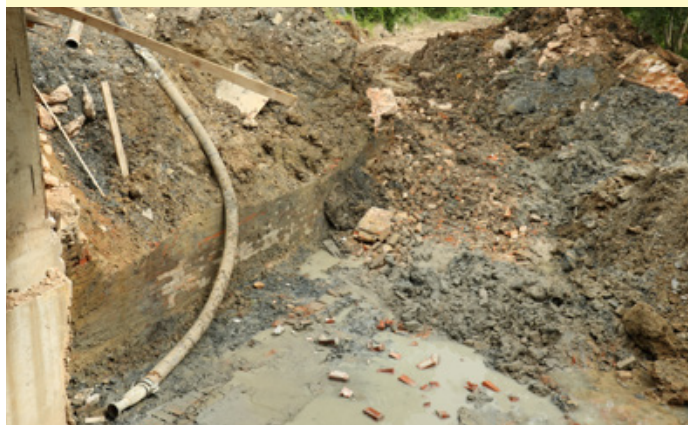
The south wall of the original bridge, shown in the top picture, would block the canal in its new position and had to be removed. The north wall (bottom picture), will be preserved but is being covered over.
