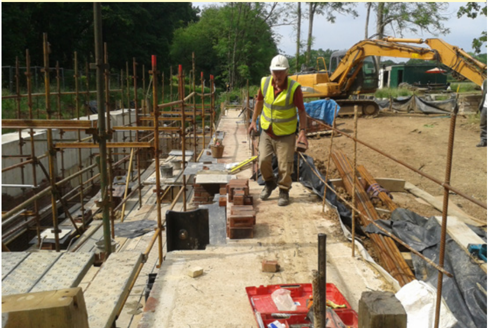
Above: the top cill of the lock. The water inlet is visible near the bottom of the left-hand ladder. Below: A view along the lockside looking north. (Geoff Thomas)
