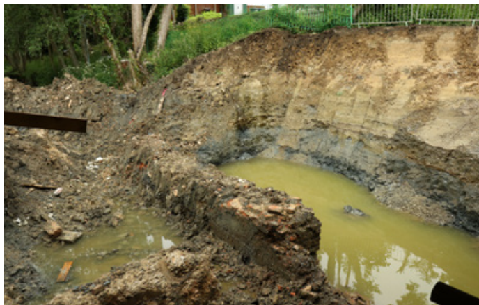
The south wall of the original bridge, shown in the top picture, would block the canal in its new position and had to be removed. The north wall (bottom picture), will be preserved but is being covered over.
