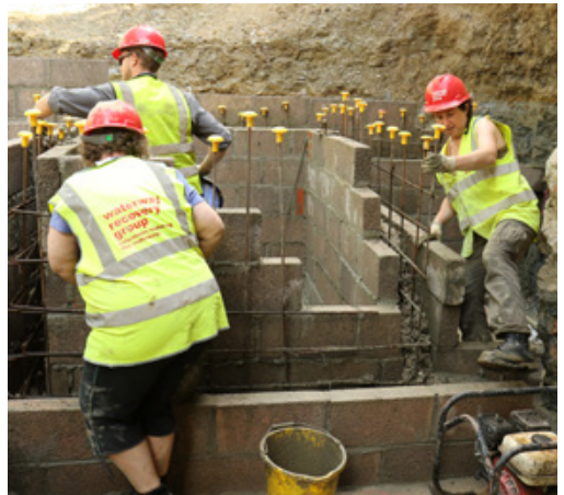
Left: In the second week, the scaffolding was erected on the north side of the bridge so that bricklaying could continue there. Right: the second week team working on the north side blockwork. (Julian Morgan)
