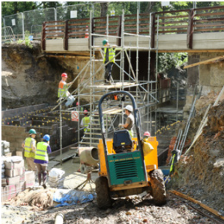
Left: In the second week, the scaffolding was erected on the north side of the bridge so that bricklaying could continue there. Right: the second week team working on the north side blockwork. (Julian Morgan)
