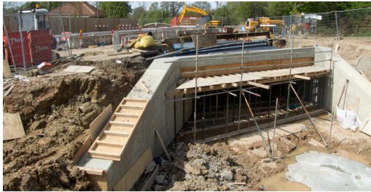
Loxwood Bridge under construction in early 2008.
