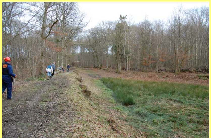
One of the Chris Richardson pictures referred to on the left, showing 'job done' in Sidney Wood. Find more at: www.myweyandaruncanal.com/sidneywoods2011.html#Final
