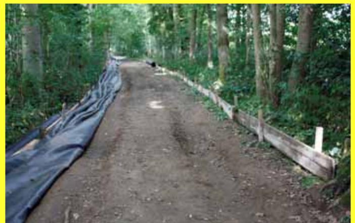
**The 4m-wide track of crushed concrete from Oakhurst Farm to GBL (photo: Janet Philips)**
