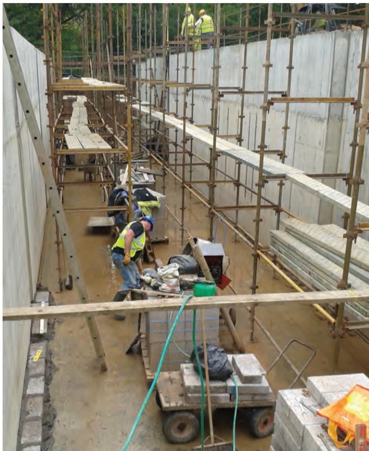
Canal Trust volunteers lay the first blocks inside the concrete shell of the new Gennets Bridge Lock, near Ifold and Loxwood.
