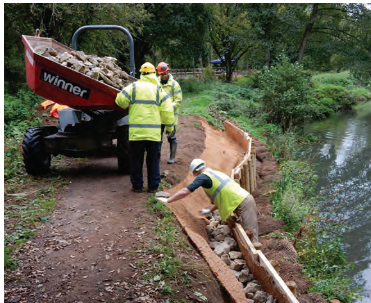
Volunteers install the new protection on the river bank.
