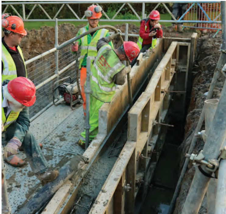
Waterway Recovery Group volunteers constructing the new slipway wall.
