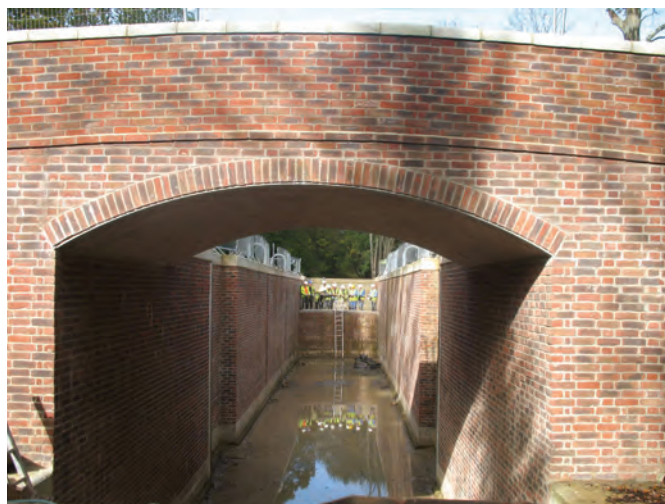
Gennets Bridge Lock as future boaters will see it - with some of the volunteer construction team at the far end.
