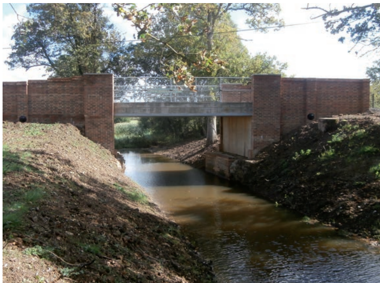
Volunteers worked tirelessly to ensure Harsfold Bridge was completed to a high standard, and to schedule.
