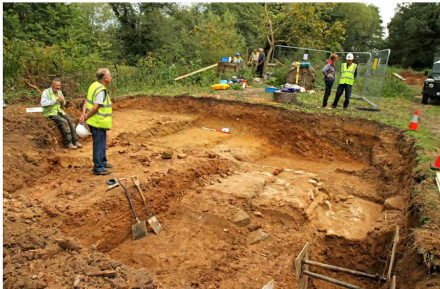
The south-east corner of the lock is visible in the centre of the picture. In the background the soil colour shows the original canal bed.
