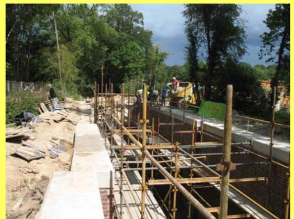
**Recent work at Southland sees the lock chamber nearing completion, with all brickwork now finished and work concentrating on the copings and training walls, ready for the gates which are now on order (Eric Walker)**
