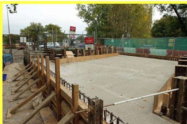
**Compasses Bridge, looking towards Dunsfold Park, showing the newly-poured concrete deck; the raised reinforcing marks the position of the parapets. (WACT picture - more at WACT website)**
