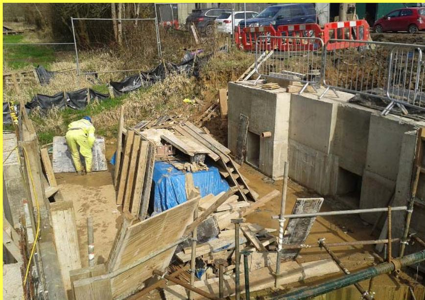
**The concrete casting for the upper offside sill at Gennets Bridge Lock is now complete. (picture by Geoff Thomas)**
