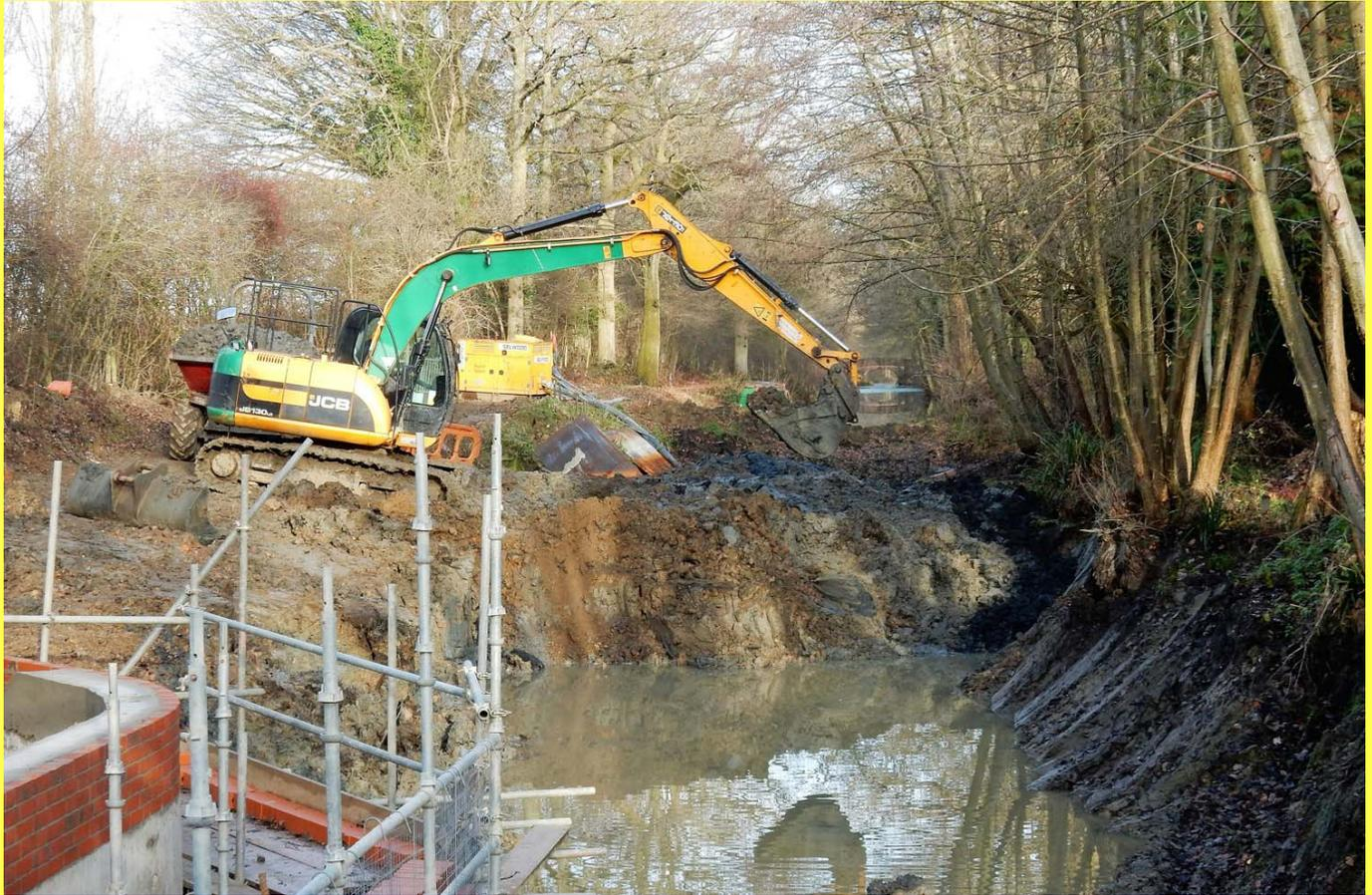
**Northern working party removing the dam at Compasses Bridge, using the Trust's excavator (Bill Nicholson)**
