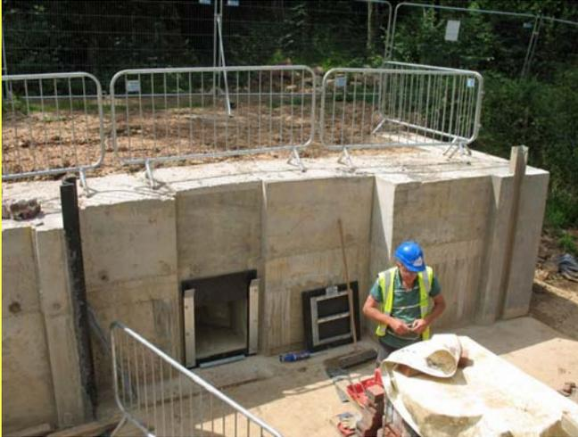
**Lock HS Sluice Blade & Connecting rod being installed**
